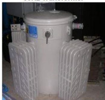
250 kVA 20 kHz transformer 330 kVA 60 Hz transformer
